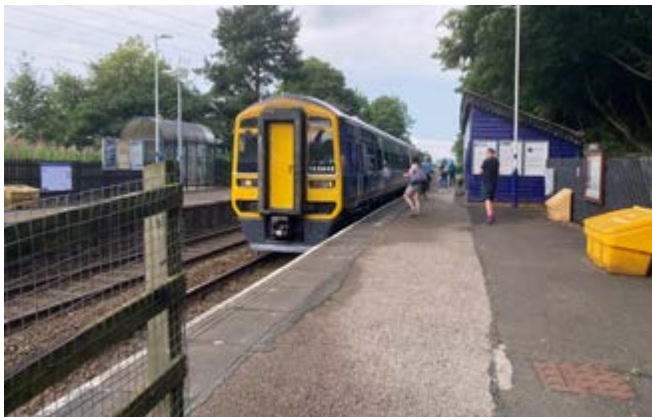
Lack of tactile paving
