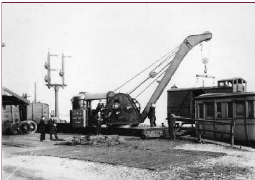
Here we see Cowans Sheldon crane number 2118, built in 1897. It was bought by the North Eastern Railway, which allocated it to the York Locomotive Department. In the photograph, the crane is seen recovering a brake van after an accident at Milford Junction in November 1907. (Joint NERA - Ken Hoole Study Centre JF Mallon Collection)
