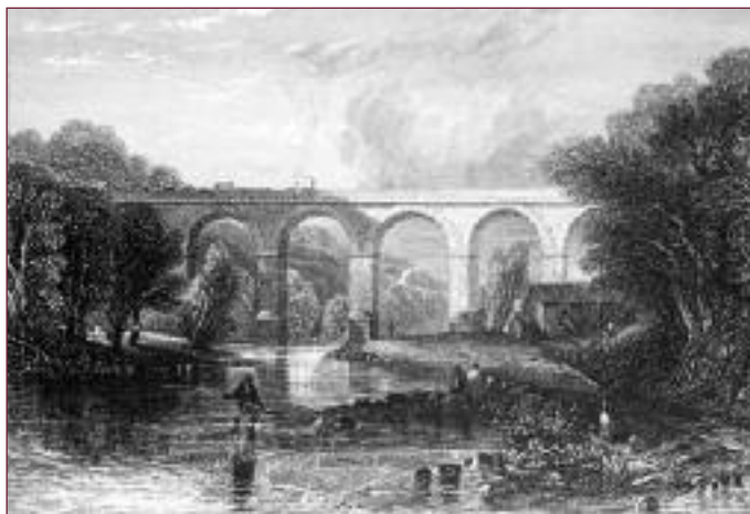
JW Carmichael's engraving of Wetheral Viaduct shortly after its opening to traffic.
