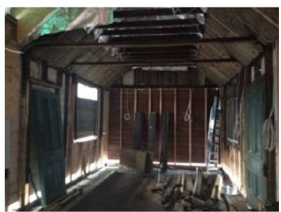
The structure was built in 1907 with external walls made of wood with wood cladding on the inside. To create a new lease of life for the building as studios fit for the 21st century much insulation has been put in place before cladding the internal walls. The windows and doors have been repaired where possible and replaced in the same style where necessary. Re-wiring and new services are being installed as we move towards decoration.
