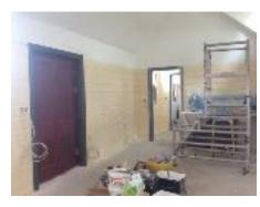
The internal and external walls, windows and doors are being painted in the same heritage colours used on the signal boxes and bridges along the line, which is cream and red.
