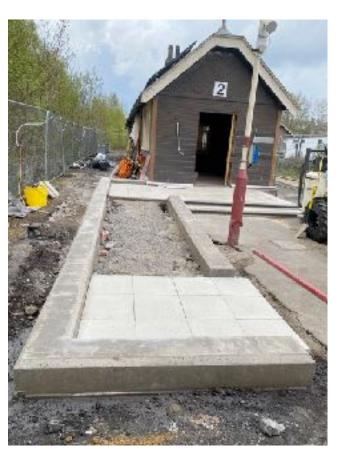
The building is of a modular structure so a door in the end of the building has been opened up as the new entrance to the waiting room. New steps have been laid and the new ramp is being constructed. A canopy is to be installed over the paved entrance area and our Hadrian mosaic will be included in a vertical position on the new railings.
