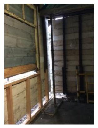
It is now mid May and we are finally almost there with the platform 2 building. The baseplate, corner posts, floor and external walls have been repaired or replaced as necessary.
